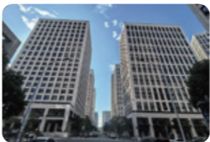
INTERNATIONAL STRAIT BUILDING
