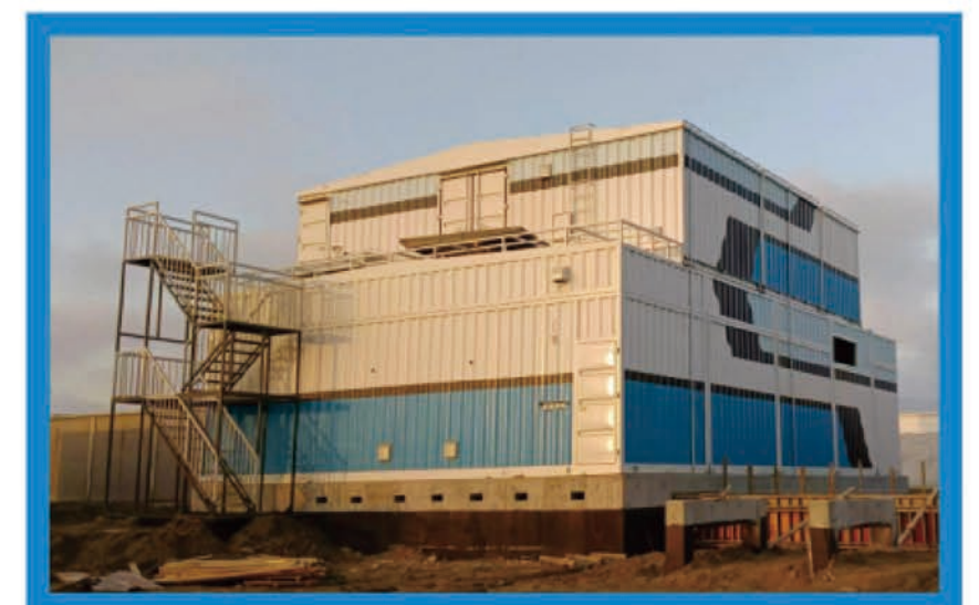
Yuanjing Sheyang 250MW 500MWh Energy Storage Power Station Project(China)
