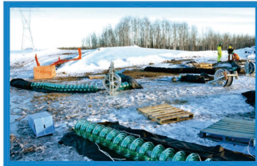
Supply of Glass Insulators for Canada's Altalink 500kV DC Project (Canada)Supply of Glass Insulators for Canada's Altalink 500kV DC Project(Canada)
