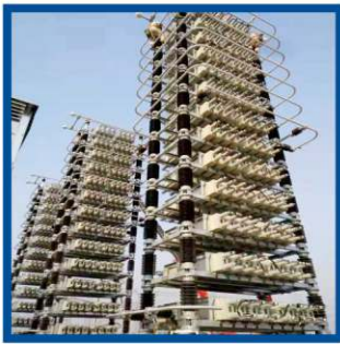
HVDC power transmission project in motija to Lahore, Pakistan
